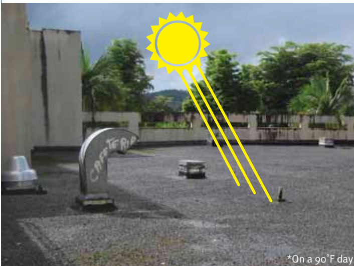
Modified bitumen absorbing sun rays 180°F
